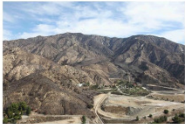
Dunsmore Canyon, San Gabriel Mtns. Photo taken shortly after the August, 2009 Station Fire; view north. Debris basin located on far right has a maximum capacity of 100,700 cu-yds. Los Angeles County Department of Public Works (LA-DPW) sediment placement site is in center of photo.
