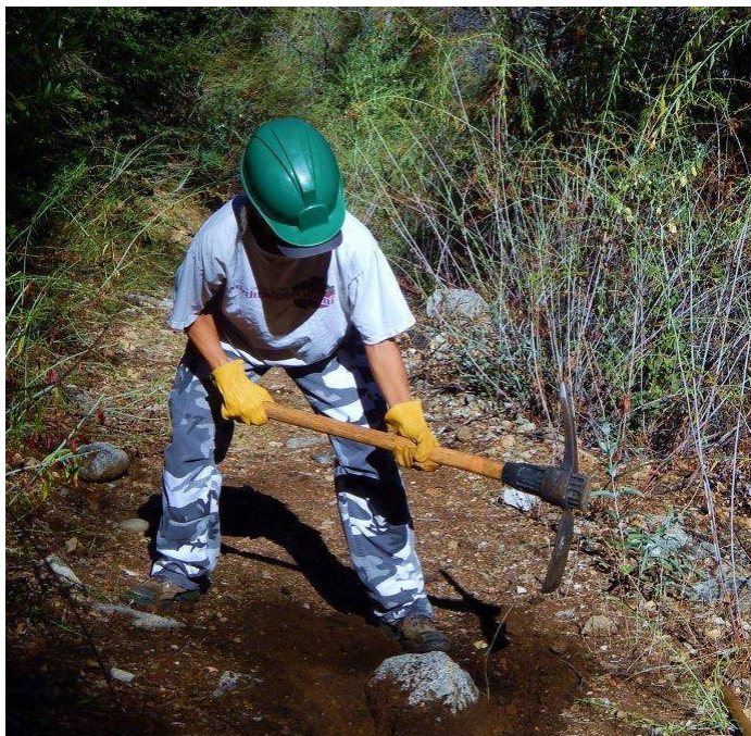
Christy removing tripper
