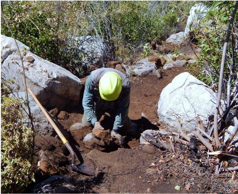
Thurman putting in steps on a small connector at the pines
