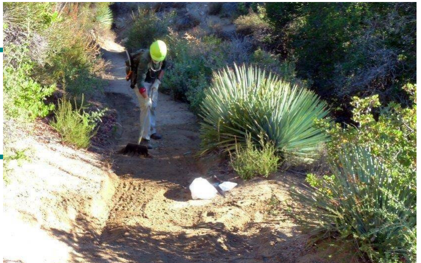
Dave working on trail near Valley Forge. Photo by Brenda Beck
