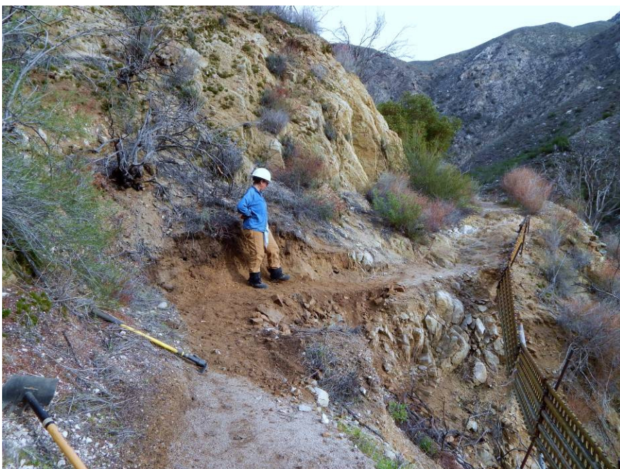
Trail Canyon Road Trail reroute, note the Marston Mat hanging in the air. by Brenda Beck
