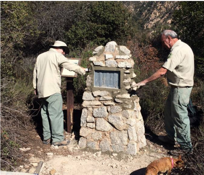
Scenic Mt. Lowe Railway restoring Sam Merrill Trail monument.
