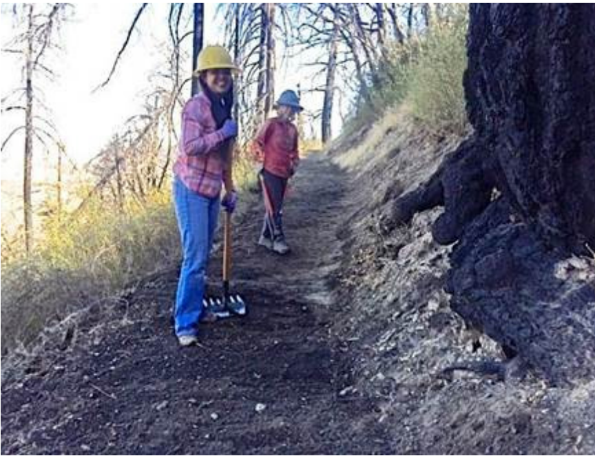
Dave Fleischman/Trail Gorillas completing the work on Station Fire Rehab at Sec D , Mt Gleason by Pete Fish
