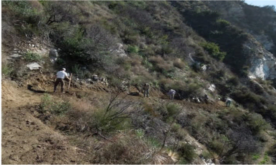
(Trail Restoration on Crescenta View Trail, December 2012)
