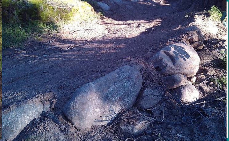
AFTER: The same trail with reinforced edges.
